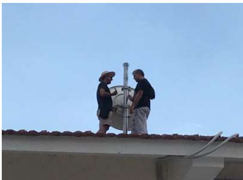
Figure 3: Installing a central node on a roof (photo by A. Voulvouli).
